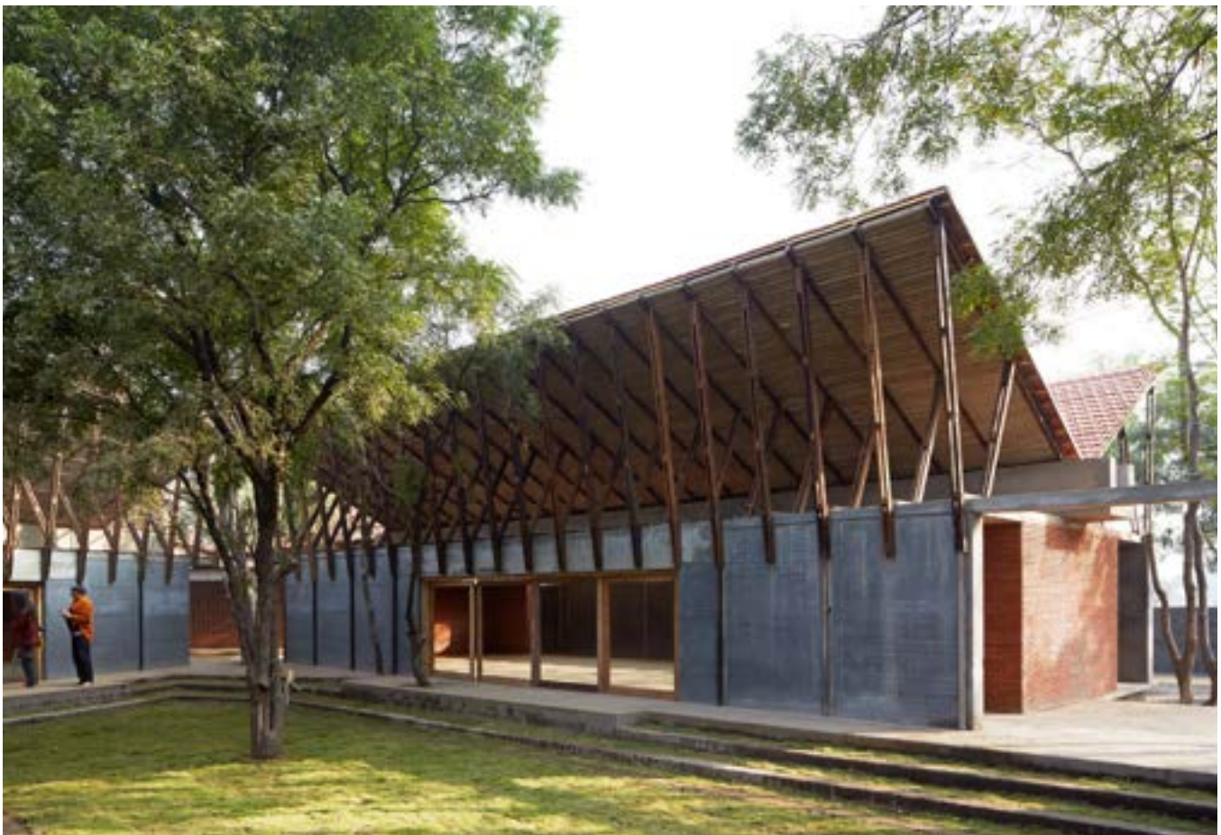
The inverted roof of Jetavana – a thoughtful blend of form and function, channeling rainwater efficiently while harmonising with the natural surroundings through low-impact design. Image courtesy Team Sankalan
